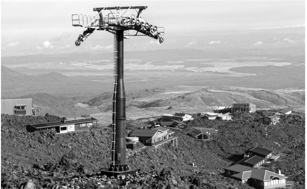
A tower in place for the new Sky Waka gondola. Photo: RAL.
