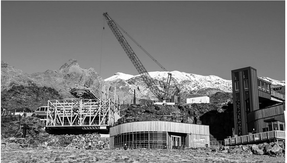
Bottom of the gondola. The lower terminal and drive station of the Sky Waka gondola were in place by early May. The building in the foreground is the Happy Valley Bistro. At the right are the access elevators. Photo: RAL.
