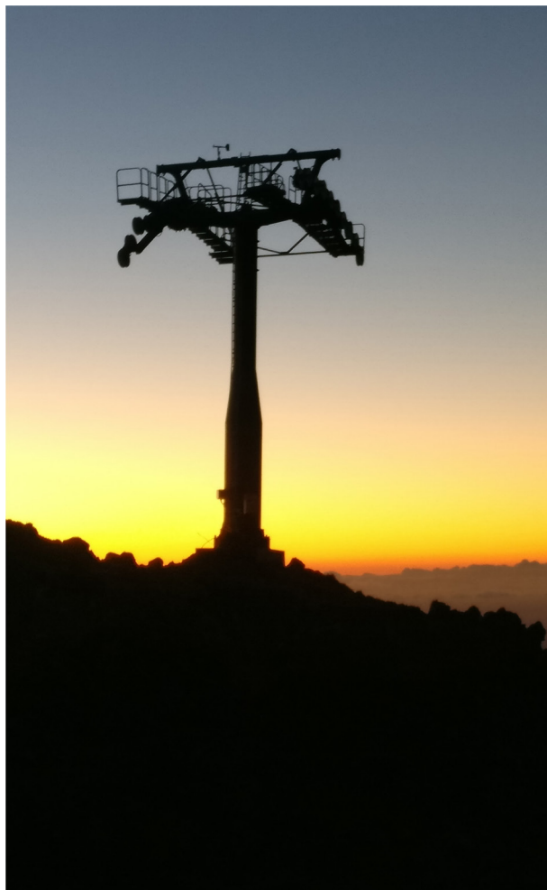
A tower for the new Sky Waka gondola which is due to open at Whakapapa later this month. Photo: Catherine Gafa.
