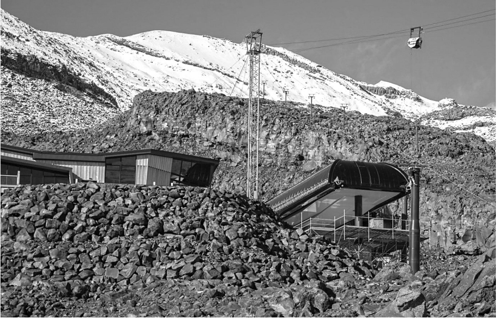
Top of the gondola. The top terminal for the new Sky Waka gondola was completed during April. Also visible is the aerial cableway carrying material from Hut Flat. The Knoll Ridge Chalet is at the left of this scene. Photo: RAL.
