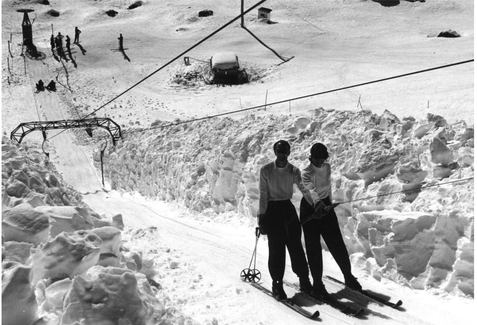
The Staircase T-bar in 1956. The n-shaped towers were replaced after 10 years by adjustable upright poles to avert this sort of digging. Photo: RSC collection.
