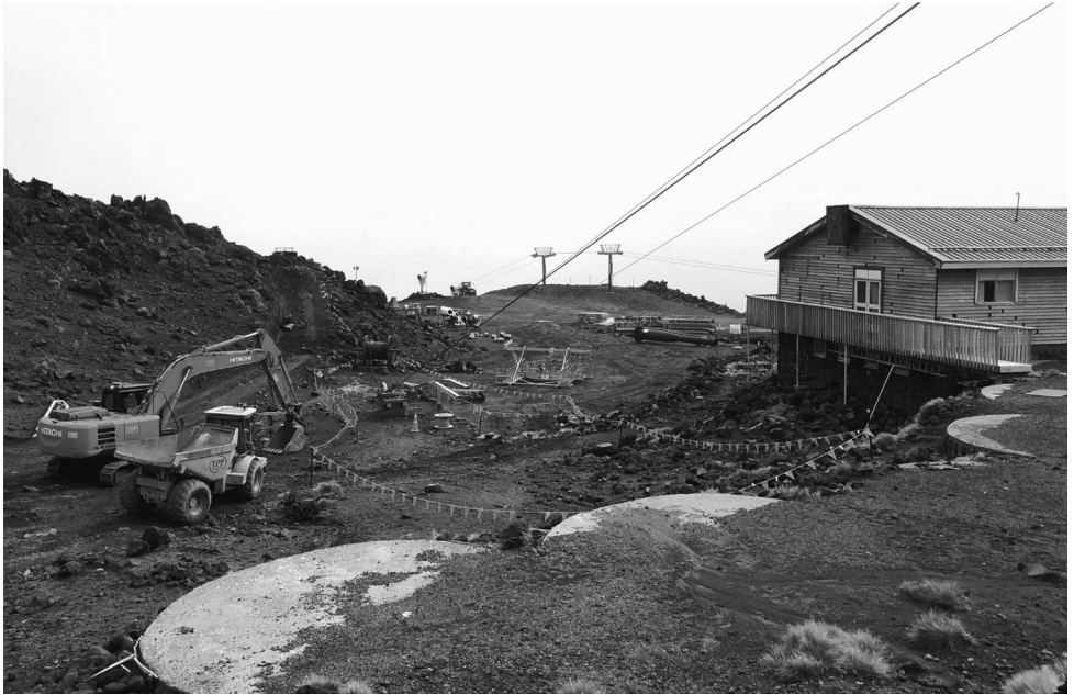
Hut Flat in March as RAL built its Sky Waka gondola. Visible is the aerial cableway (flying fox) that carried tons of cement up to the tower sites. The cement was driven by tractor up the Rockgarden and then transferred to the cableway. Photo: Dan Paine.
